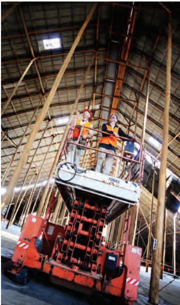
ABOVE: Conservation works underway in the Murtoa Stick Shed in 2010 - 11.
