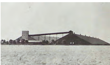
ABOVE: Murtoa Store No 1 (left) and No 2.
