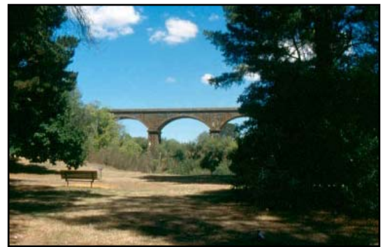
View of viaduct from Botanic Gardens
